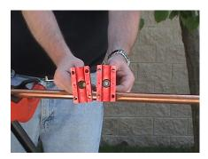
Apply the gasket sealant to both body halves and allow 1-2 minutes for dry time.
