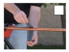
**Step 1**Before installing the Add-A-Valve®, clean the copper tubing with a fine emery cloth until the copper tubing has a bright, shiny finish.
